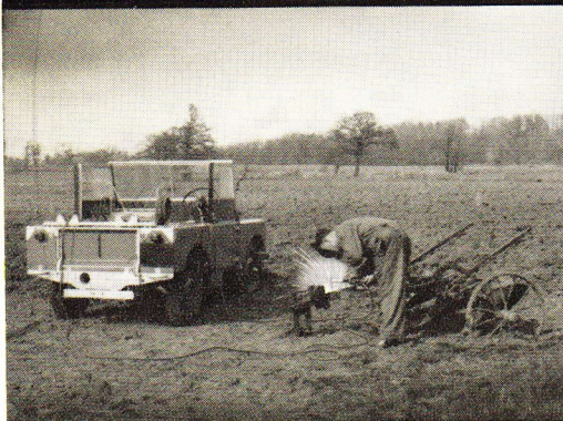
The Land-Rover mobile welder takes the power to the job.
