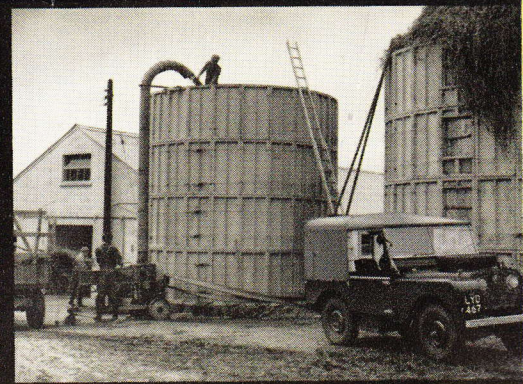
The Land-Rover provides power for the Silo lift.
